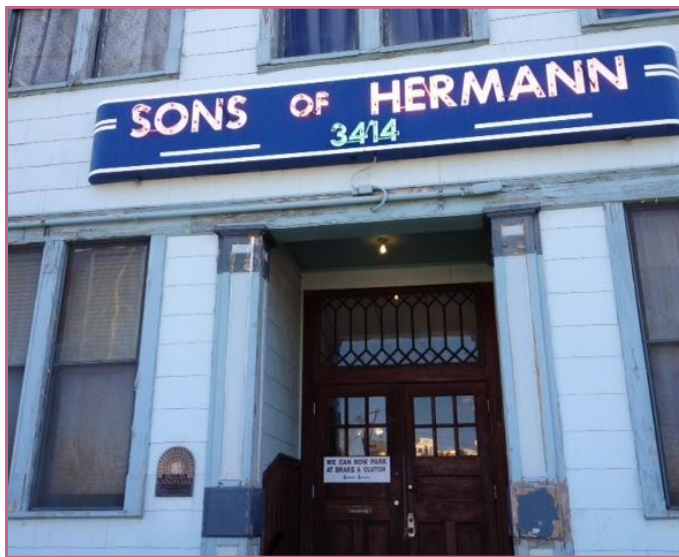
The Sons of Hermann site, completed in 1910, was built as a temporary facility but later found use as a dance hall, bowling alley and meeting place.
