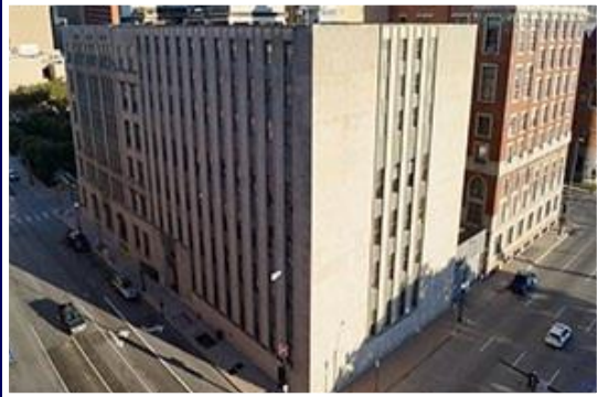
Dallas County Records Building Complex
