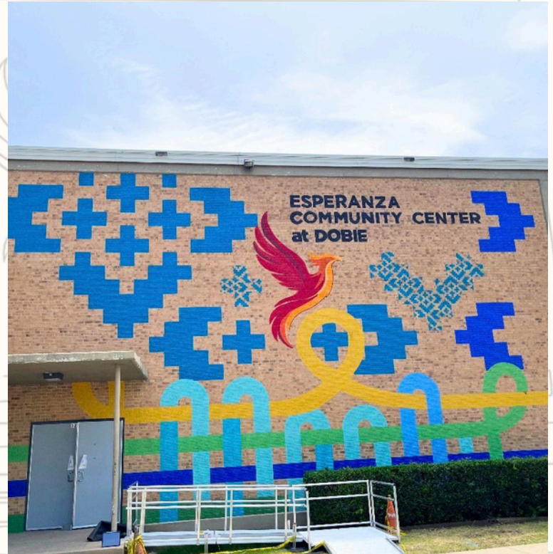
The Esperanza Community Center featuring the new murals painted on the outside of the gym.
