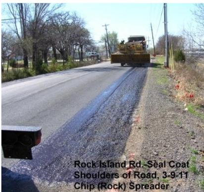
Rock Island Rd.-Seal Coat Shoulders of Road, 3-9-11 Chip (Rock) Spreader
