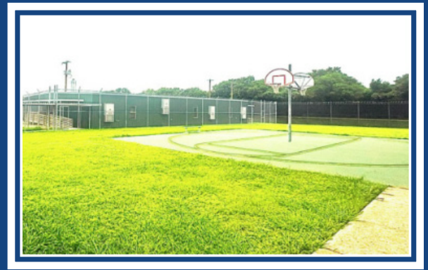
Part of the finished school at Medlock
