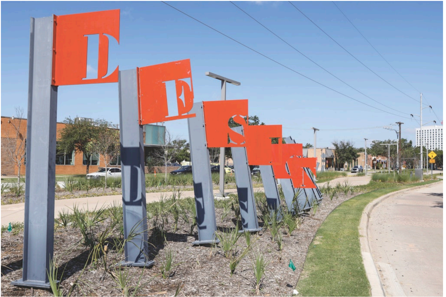
I-beams line the newly open Hi Line Connector trail in the Design District. Thanks to a $15 million upgrade, the formerly dank and unsafe highway passageway linking Victory Park and the Design District features colorful lighting, expanses of white rock and helpful signs. Soon to be activated are traffic signals designed to better separate pedestrian and car movements. (Photos by Elías Valverde II/Staff Photographer)
