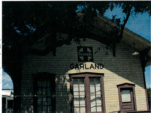
In its heyday the . The depot was the home of the Santa Fe railroad.
