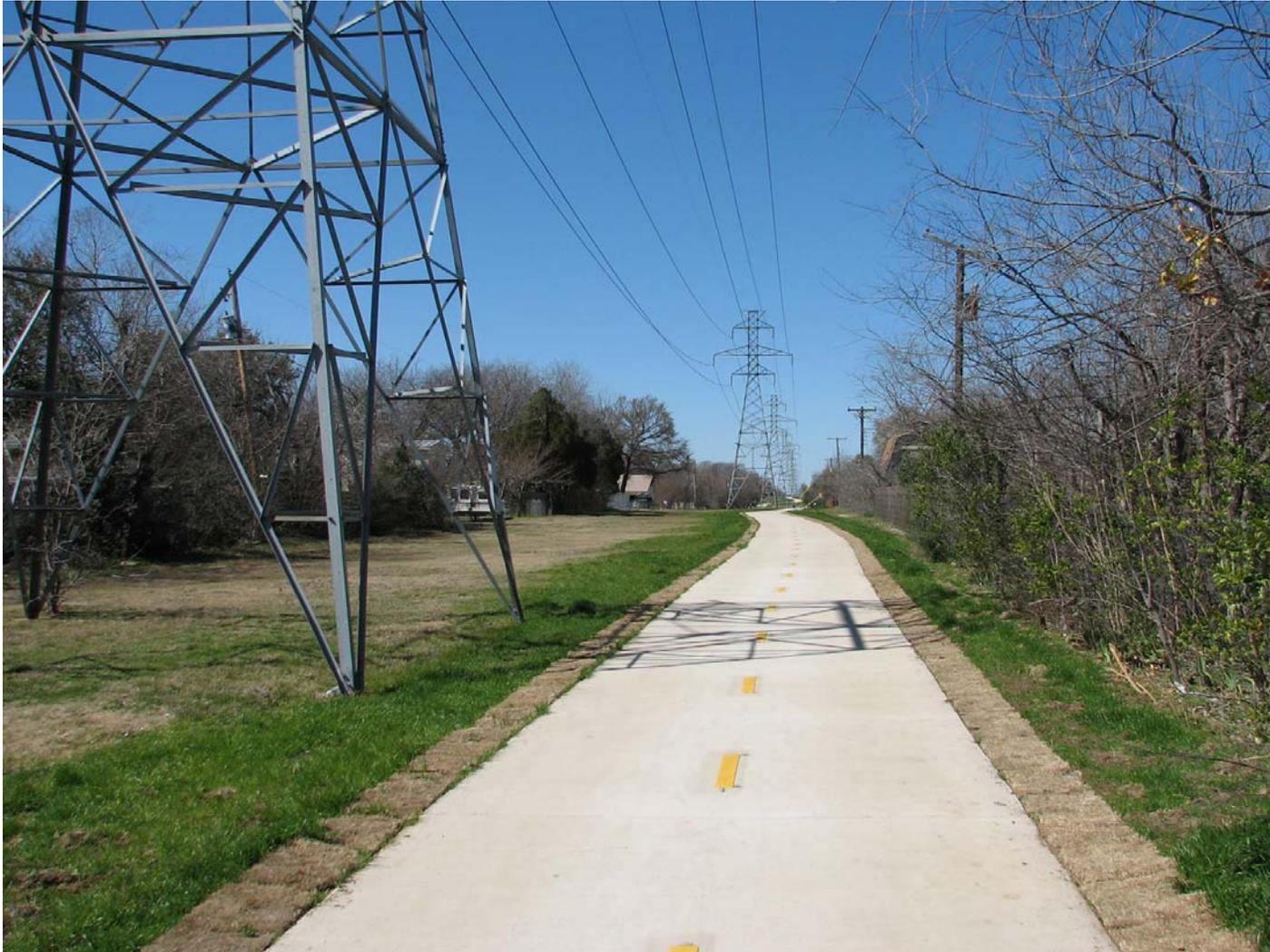
*This is an example of a newly developed 12' wide concrete trail located along a utility easement in North Richland Hills, TX.*
