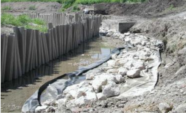
Riprap Installation
