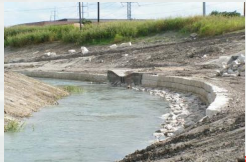
Cut Stone Wall Facing Downstream
