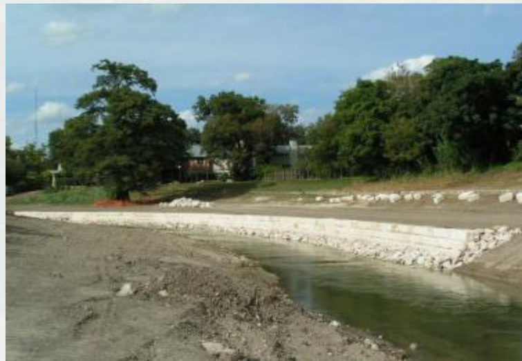
Cut Stone Wall Facing Upstream
