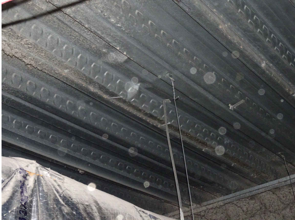
46.1 REPAIR AND REPLACE BENT CORRUGATED METAL DECK
