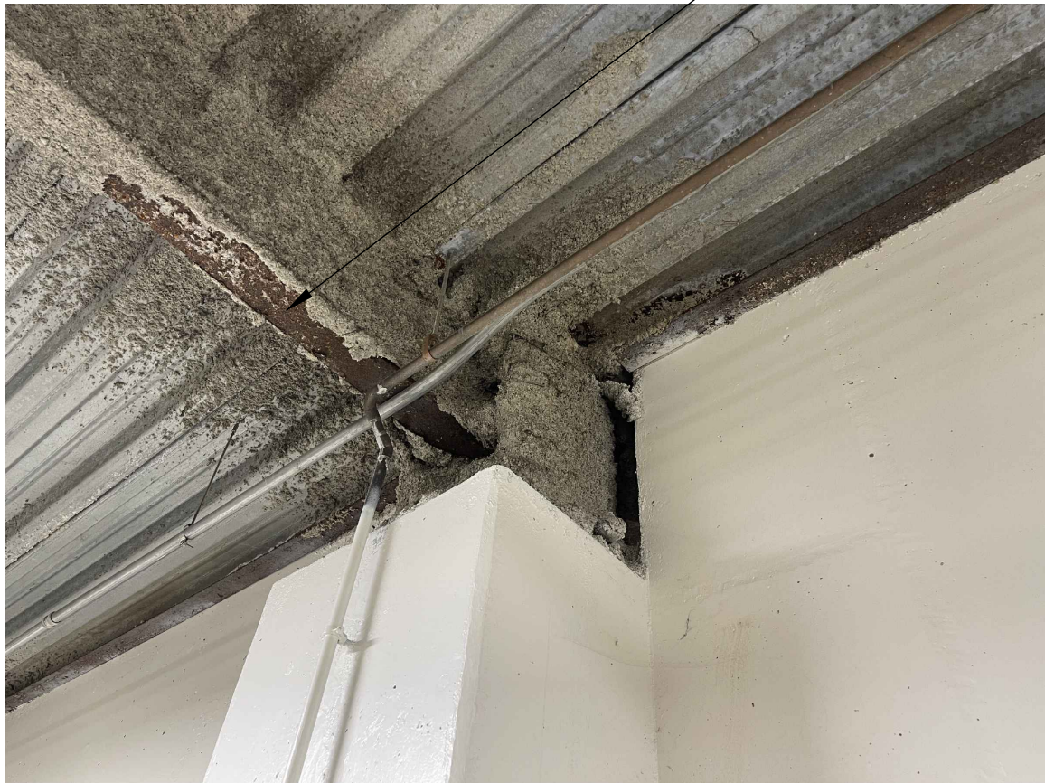
46.3 STEEL BEAM-CLEANING, COATING AND INSTALLATION OF FIREPROOFING
