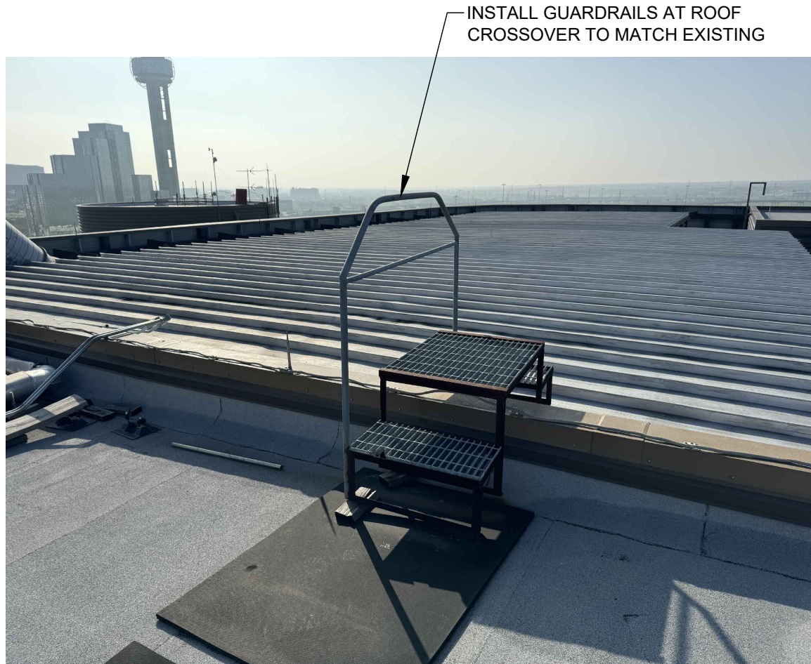
INSTALL GUARDRAILS AT ROOF CROSSOVER
