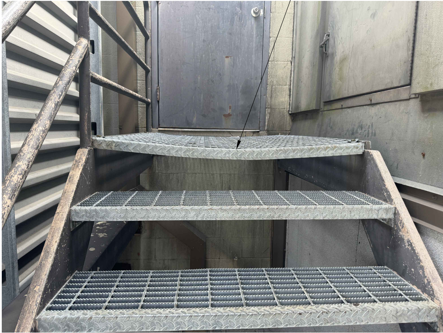
45.8 REMOVE AND REPLACE BENT GRATING LANDING AT STAIRCASE TO ELEVATOR PENTHOUSE
