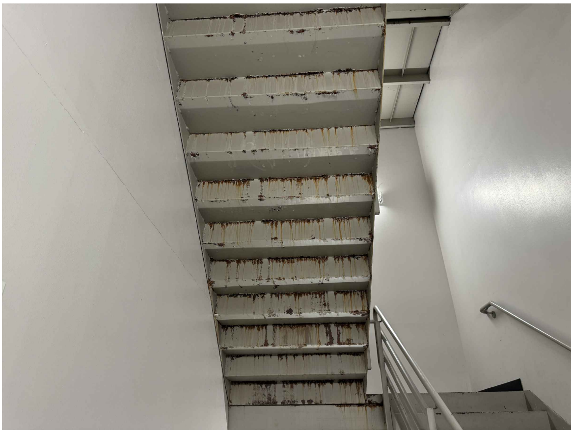
ABRASIVELY CLEAN AND COAT WITH CORROSION INHIBITING PAINT
